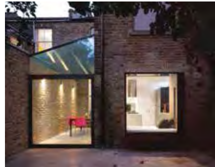
An angled glazing providing daylight to the extension without overshadowing the neighbor by Platform 5 Architect
